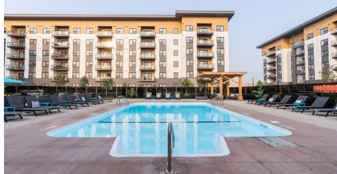
Vibe Apartments 90 Arbour Lake Hill NW, Calgary
